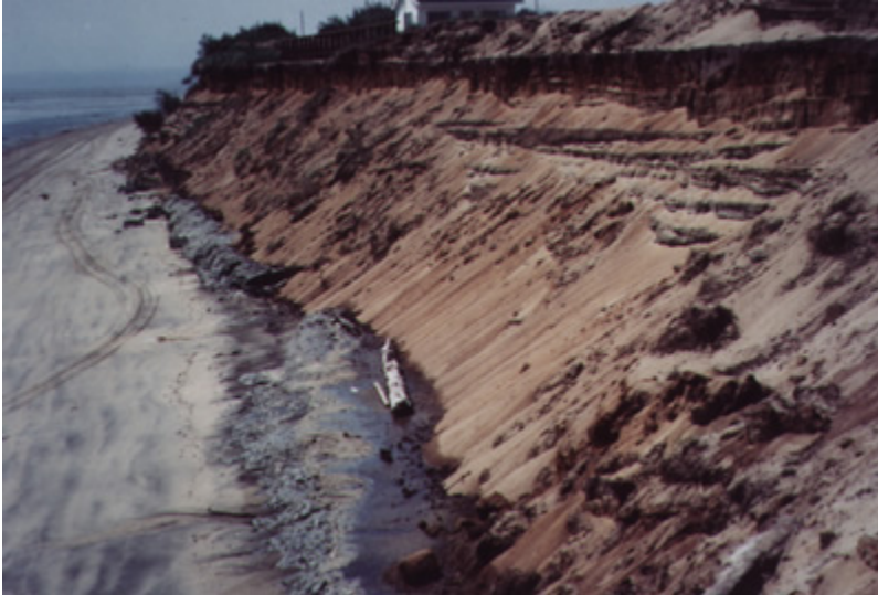
Photograph G. Pointe aux Outardes, Quebec Source: J.-C. Dionne.
